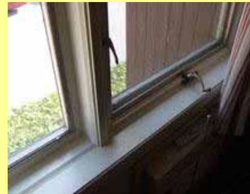
View of the window frames
