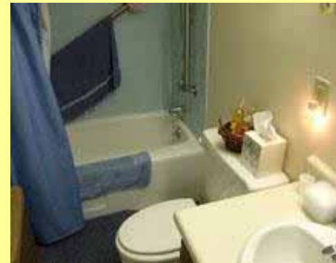
Typical view of bathroom finishes
