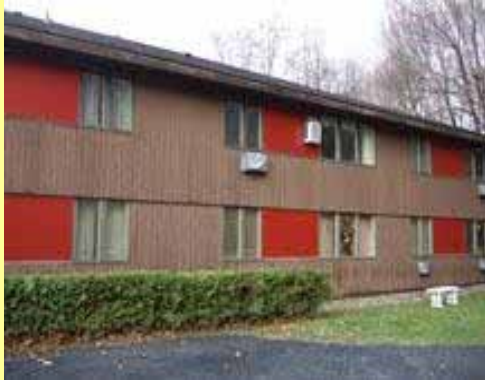
Typical view of the exterior siding
